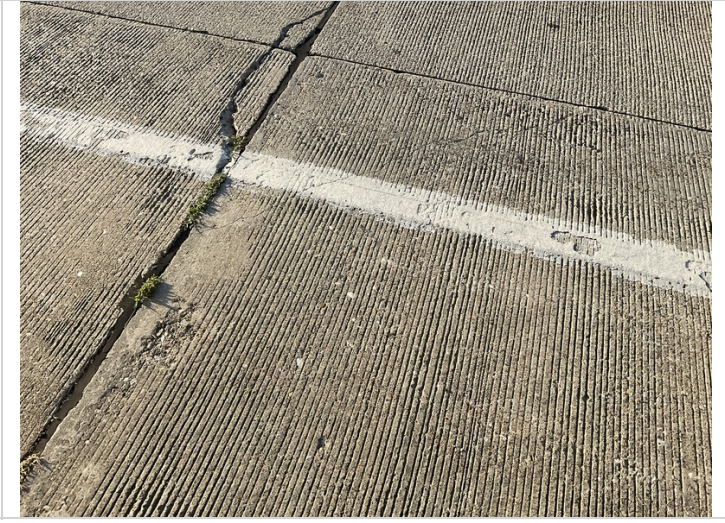
07/22 bent 6 large cracking in deck
