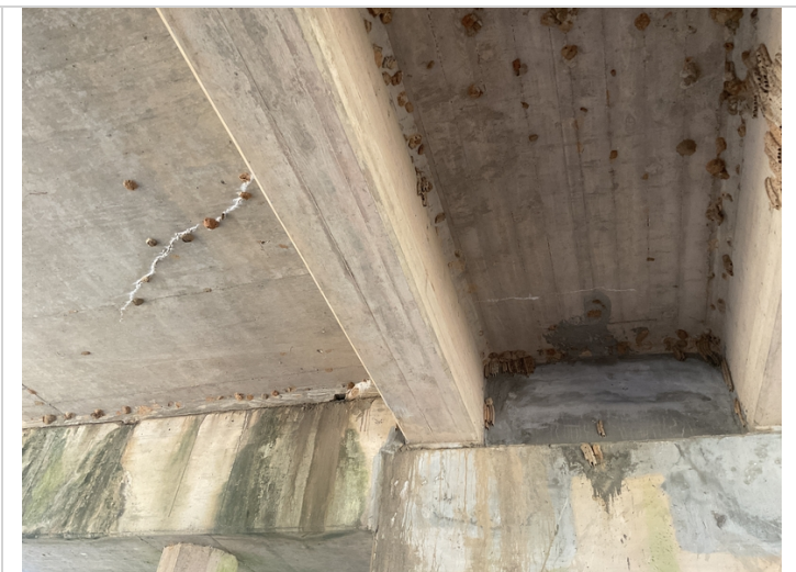
07/22 efflorescence in span 2
