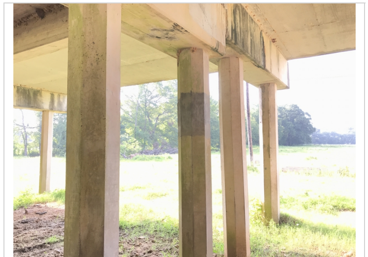
Bent 3 pile 6 patch
