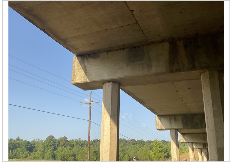
07/22 bent 6 top of right side outer cap has spall area
