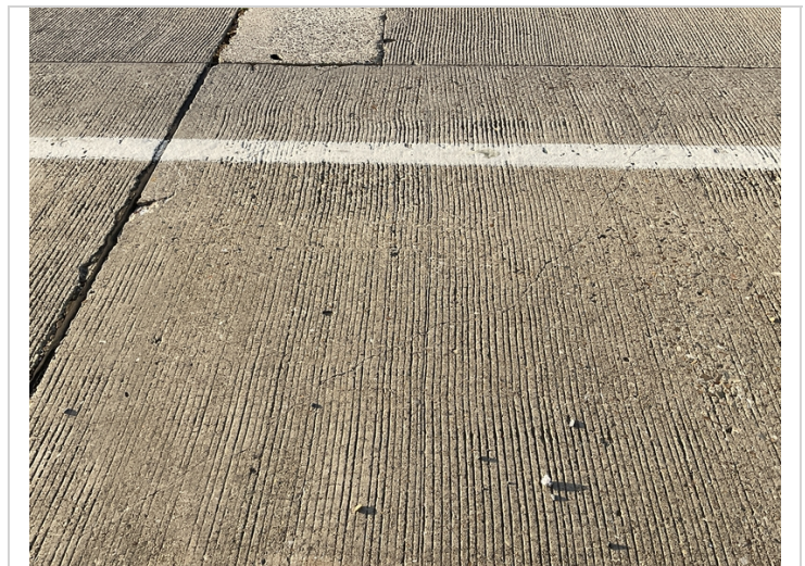
07/22 cracking in deck
