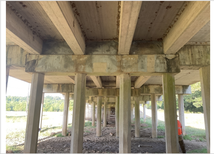
07/22 bent 7 both ends of center cap have spalls in top corner
